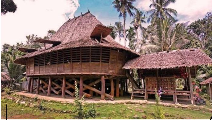
House in Nias, North Sumatera, add cross bracing to withstand frequent earthquake shaking.
