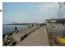
Break water to protect the port
