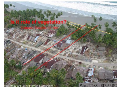
Damaged houses struck by a 3-4-m-high tsunami; some of the houses behind the coastal forest were saved (Sirambu, West Nias)
