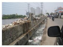
The dike to protect the settlement
