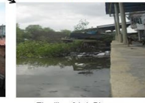
The dike of Asin River
